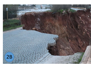
Google image showing the geology of the Estremoz Anticline (1) and the landslide of the quarry slope on November 15, 2018, with a length of 100 meters (2A), which was located next to the M255 municipal road, causing it to collapse (2B) and deep cavities with dangerous vertical slopes, interspersed with increasingly high and visually striking rock heaps Anticline (3).
