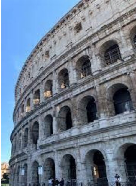
Figure 3. Image of Colosseo, also known as Anfiteatro di Flaviano, using Travertine in its structure.
