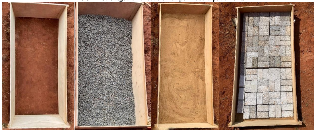
FIGURE 3. Stages of execution of permeable pavements
