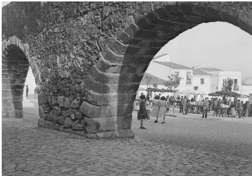
Figure 1. Former market in Largo do Chão das Covas (1949 to 1960). Photograph: David Freitas. © Évora Municipality Photographic Archive.
