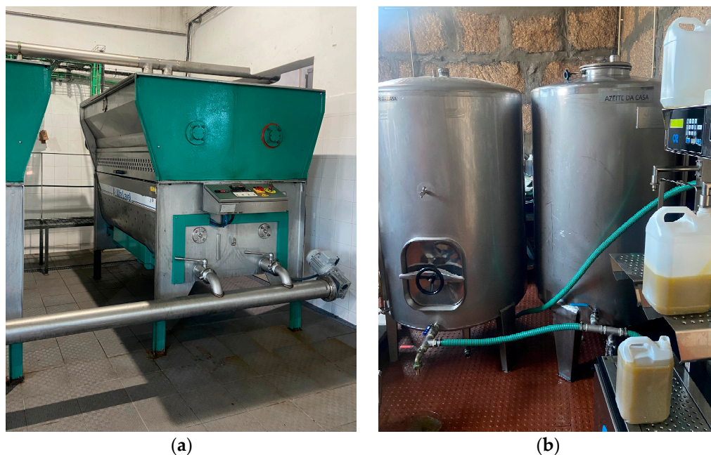
Figure 4. Production line equipped with stainless steel tubes versus plastic hoses. Photo (a) shows steel tubing, whereas (b) shows plastic hoses.
