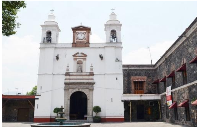
Figure 31. Facade of the Inmaculada Concepción church on the left and on the right the "Juventino Rosas" House of Fine Arts.
