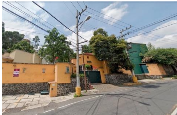
Figure 40. Santa Teresa walls in the Bosque Santa Teresa horizontal condominium.
