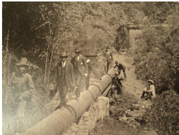
Figure 20. Photograph showing the piping system of the 1 st Dinamo and a group walking on it.
