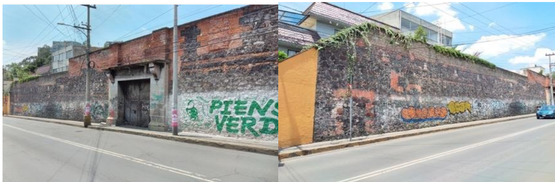
Figure 38. Santa Teresa Northern walls.
