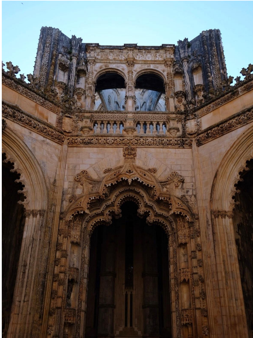
Figure 2.1. Facade and ornaments with orange patina at the Imperfect Chapel, Batalha Monastery
