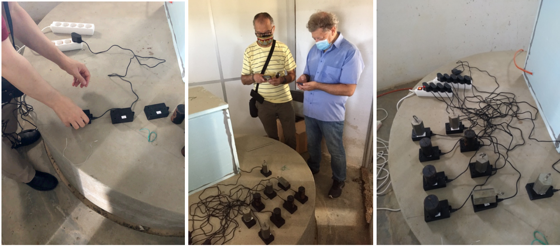
Figure 57 - Installation of sensor prototypes at MITRA station
