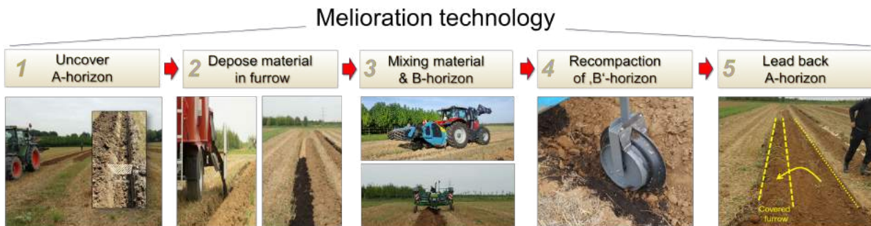
Figure. 2: Phases of the Soil 3 melioration process and selected photos of the technology from the preliminary tests for tool selection and design.
