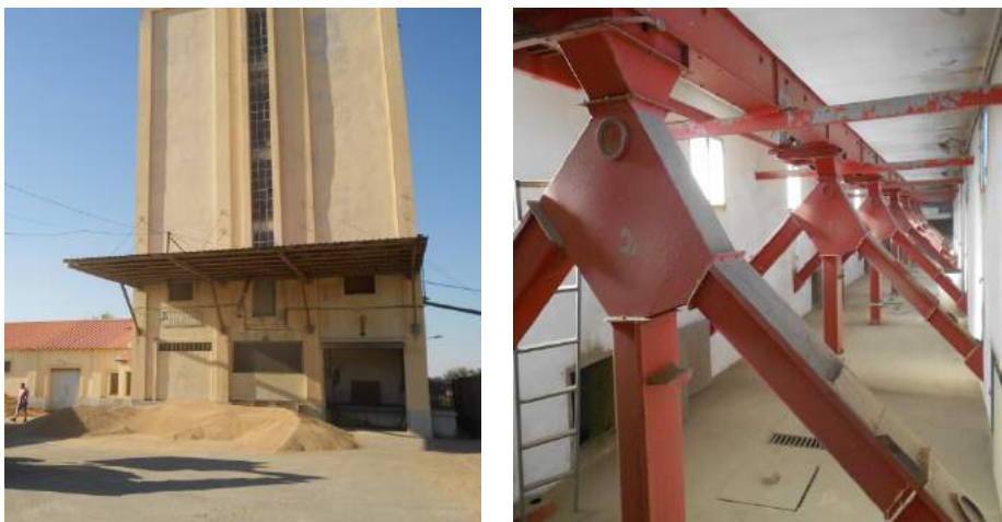
Figure 3. Detail of hopper area and upper horizontal belt conveyor and distribution tubes in D 5 silo at Manganeses de la Lampreana, Zamora
