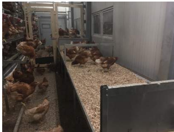
Figure 9: Rear view of one of the two units as installed in the pilot farm.
