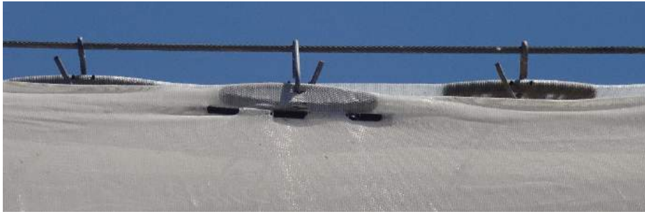
Figure 2 Special Net-to-Cable connector
