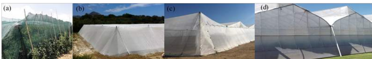
Figure 1. Local-type and standardized nethouses: (a) pitched-roof, wooden (Kittas and Katsoulas, 2018), (b) flat-roof, steel (Skytop, Greece), (c) duopitch, steel (Polysack, Israel), (d) gothic (Arrigoni, Italy)
