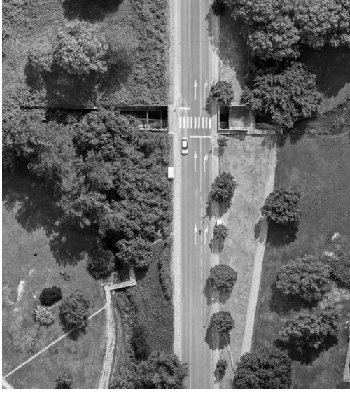
Fig. 13 - Aerial view of the wooden bridge and the water passage (Brito2020)
