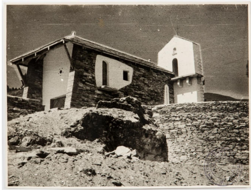
Fig. 5. Chapel for FENOSA in Erberdeiro (Chantada), 1955
