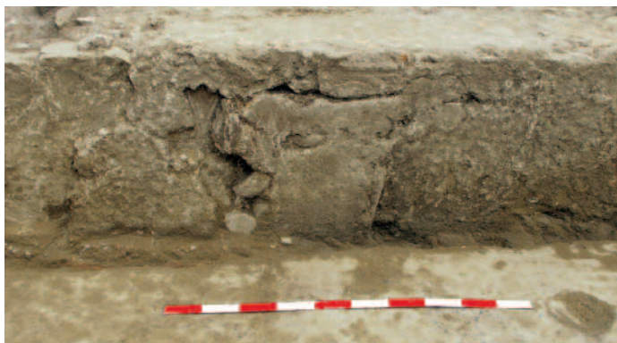
Fig. 4. Northern wall in the stibadium room [UE40] with marble slabs removed.
