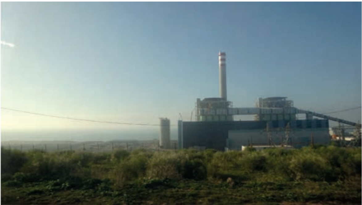
12. View of the new thermoelectric complex located south of Safi © João Rocha
