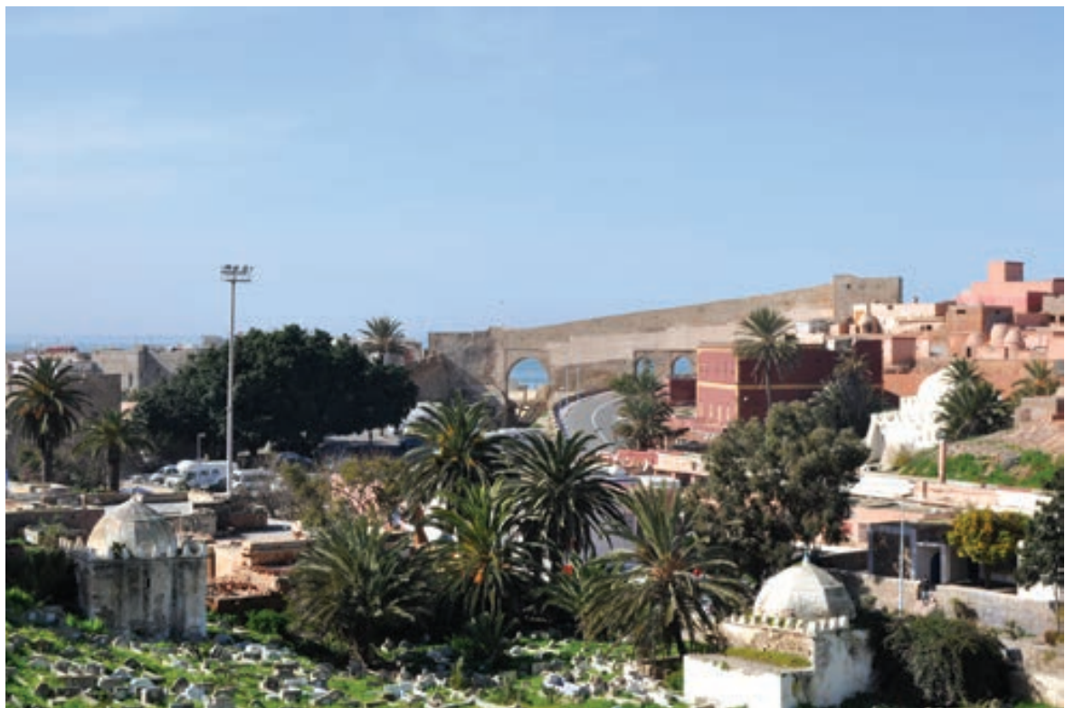
5. View of albarrran tower from the Sea Castle © João Rocha 5. Vista de muralha e torre albarrran do Castelo do Mar © João Rocha
