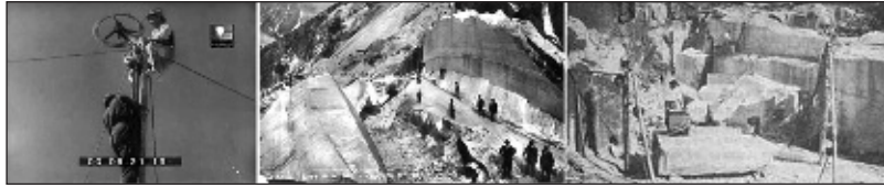
Fig. 4. Still images from the films showing the helical wire saw in use to cut marble blocks in both Italian and Portuguese quarries in the 1930s.
