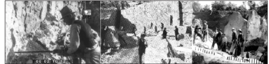
Fig. 3. Still images from the films showing the pneumatic drill or jackhammer in use in both Italian and Portuguese quarries in the 1930s.
