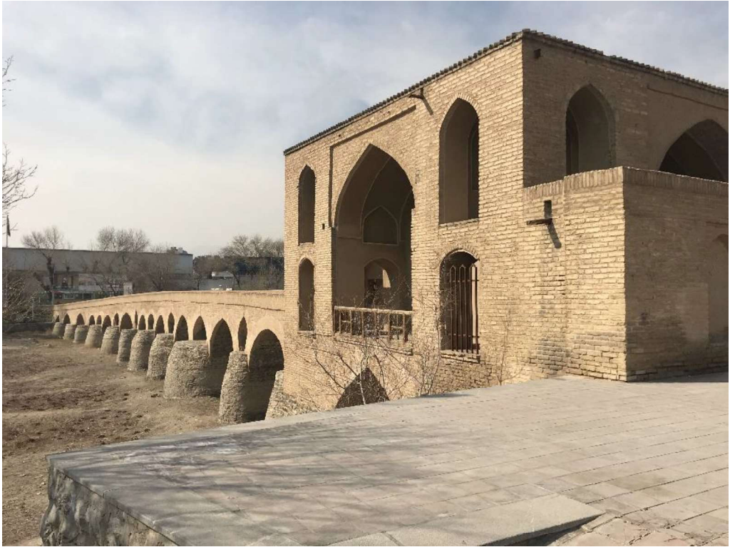
Fig. 45: The three-store structure of the bridge, Author.
