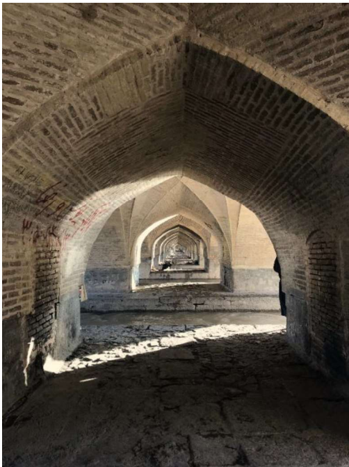
Fig. 62: The arches under bridge, Author.
