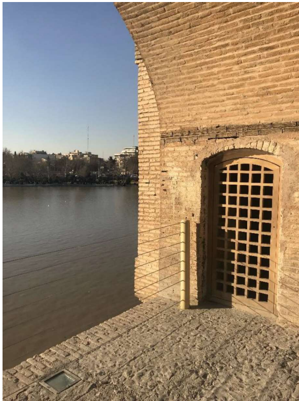
Fig. 60: Entrance of the one room on bridge, Author.
