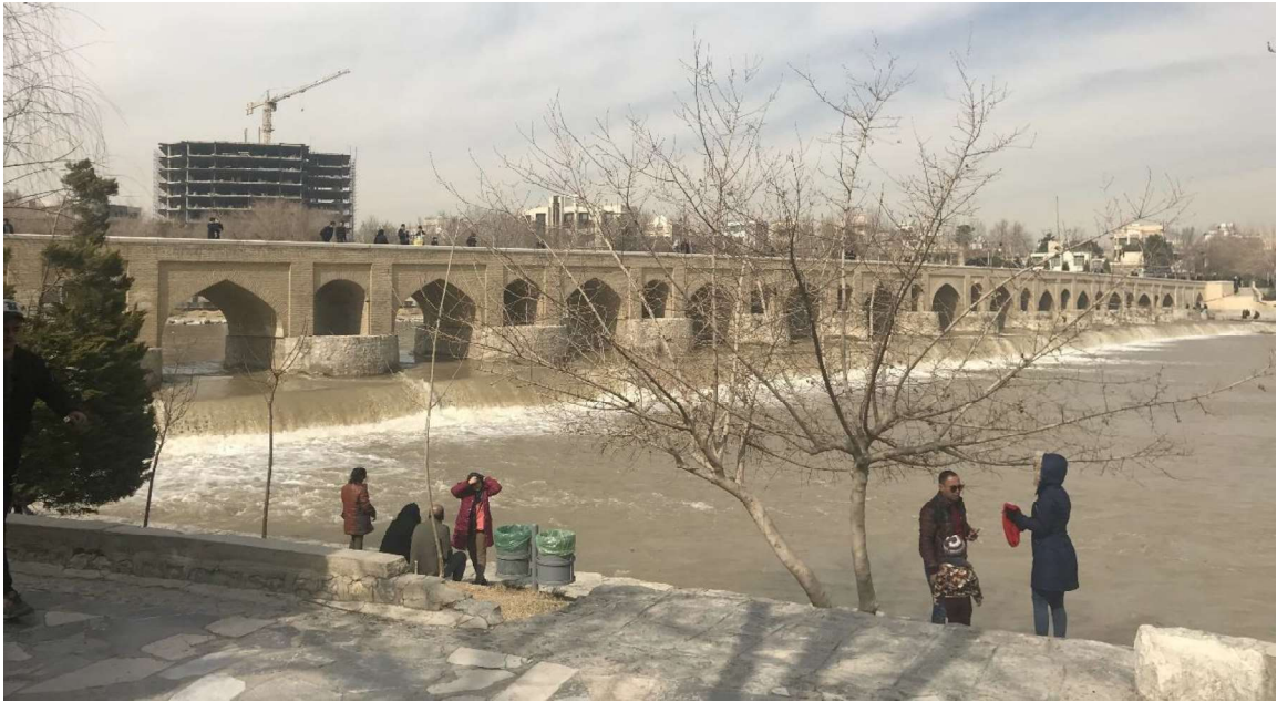
Fig. 48: Picture of the Marnan bridge, Author.
