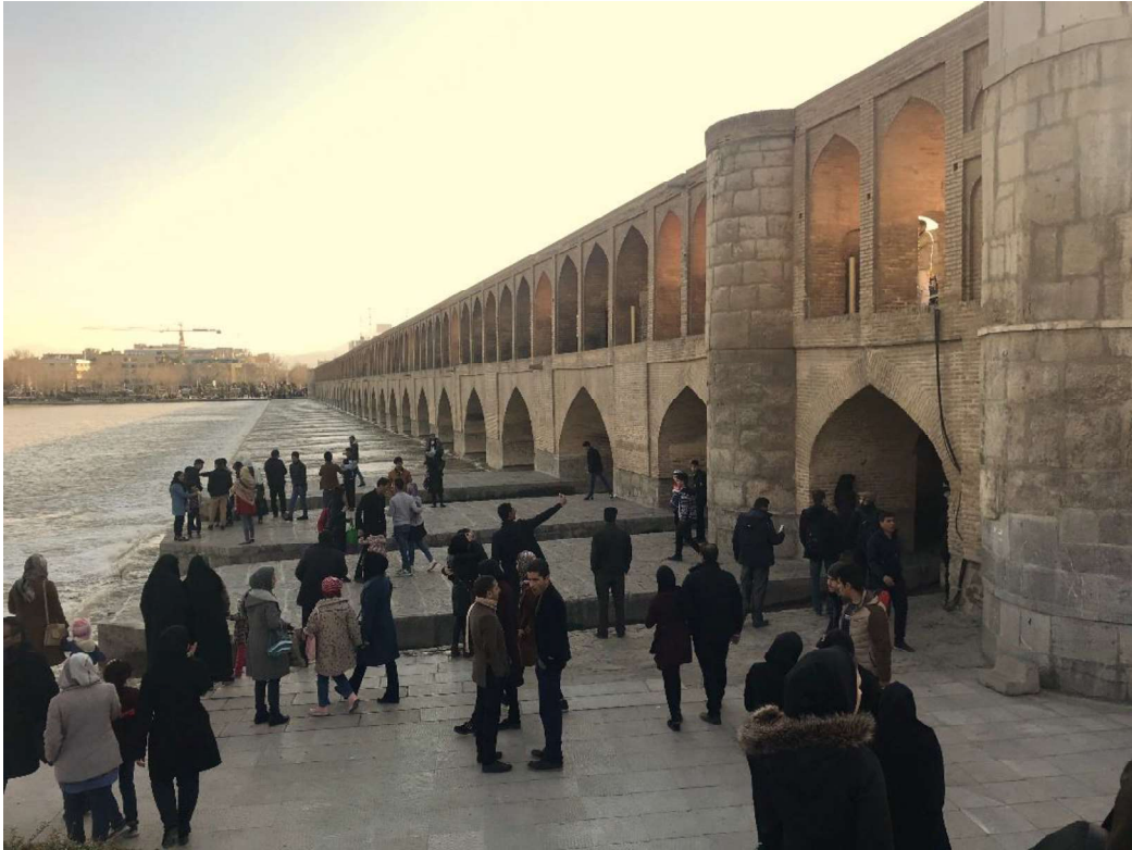
Fig. 61: The columns of the bridge, Author.
