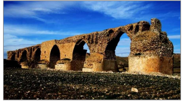
Fig. 13: Kashkan bridge, www.flickr.com, 2009
