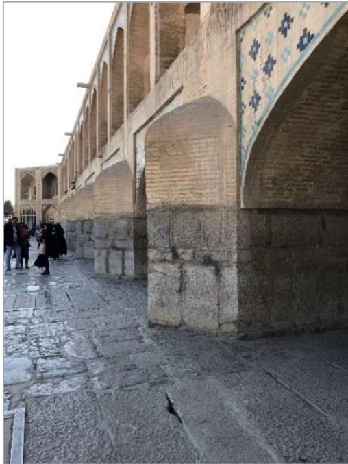
Fig. 4: Breakwaters of Khaju bridge, Author
