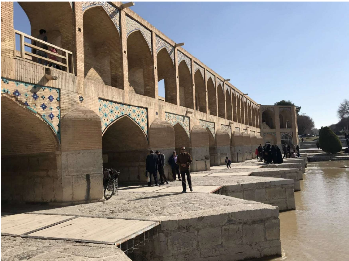
Fig. 82: The used materials (Brick and stone) are visible in this picture, Author
