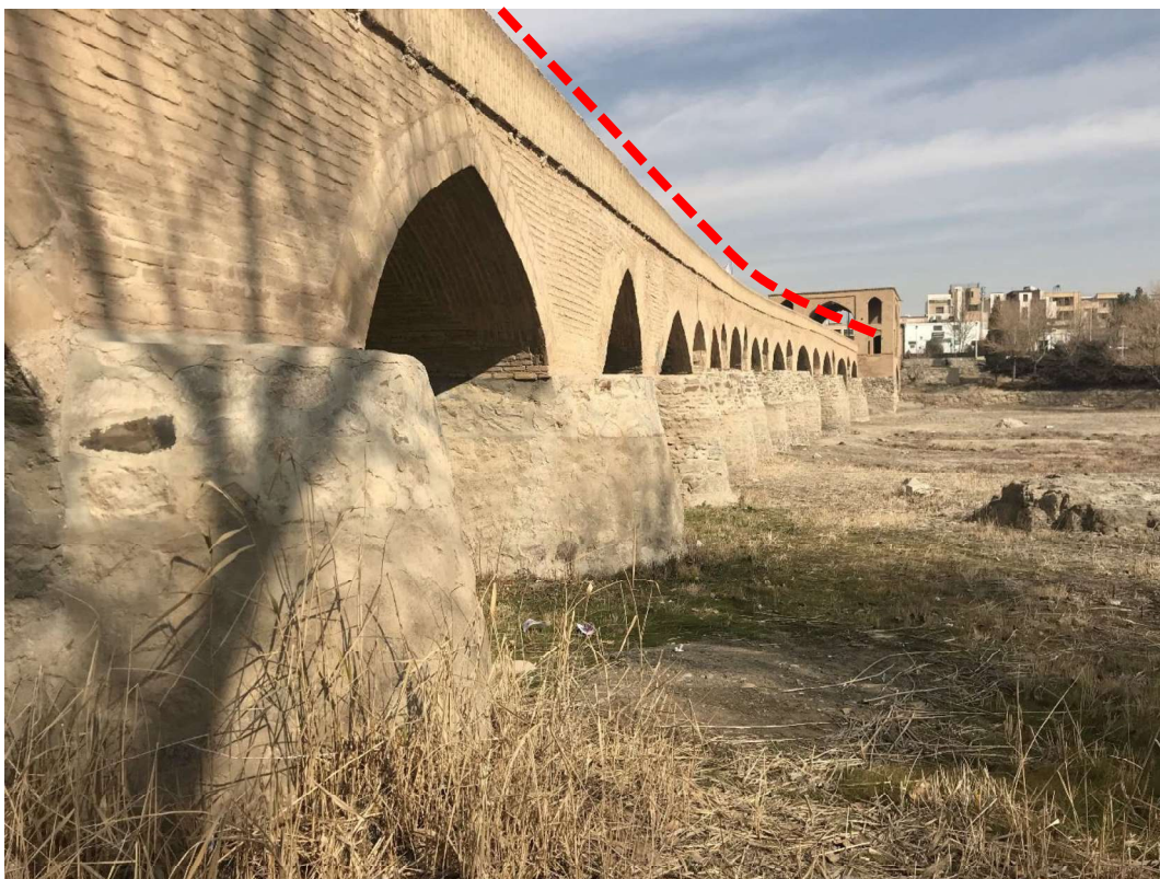
Fig. 43: The parabolic form of the body of bridge is visible in this picture, Author.
