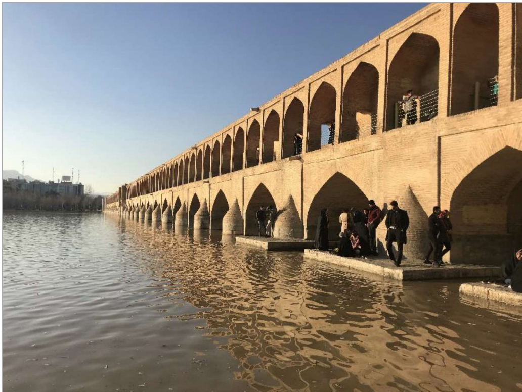
Fig. 6: Breakwaters of si-o-se pol, Author
