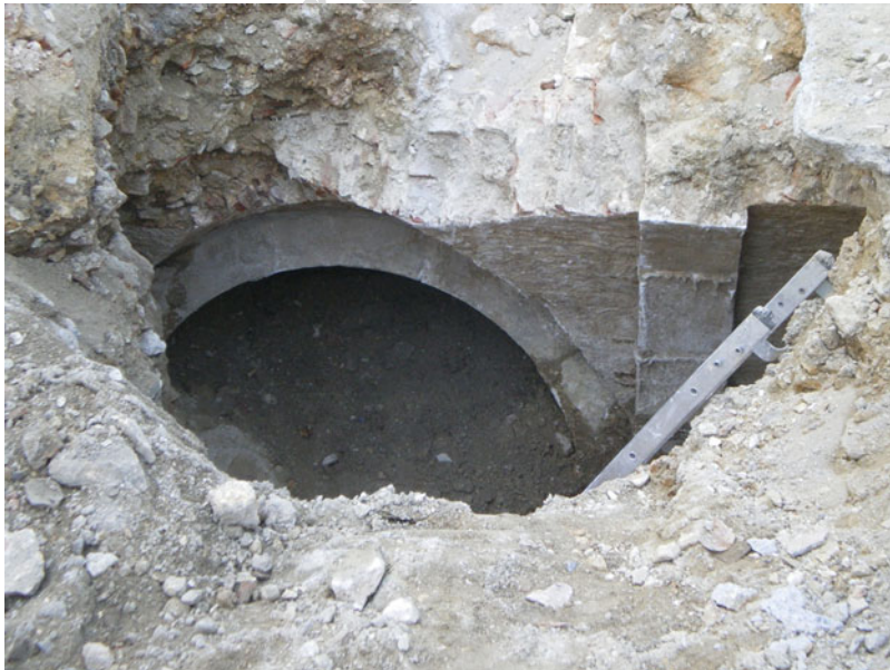
Fig. 5.25 Picture of the structure (ceiling/tunnel?) found during construction work in the area of the geophysical survey. The structure is filled with sand, rocks, and dirt. The dimension of the structure can be appreciated by comparing its size with the upper part of the ladder in the right portion of the picture
