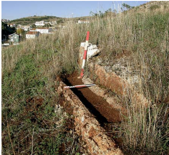
Fig. 5. Section of the Roman aqueduct (commonly called as Amadora aqueduct), in Gargantada zone, ca 700 m south of Carenque (photo José Manuel de Mascarenhas).
