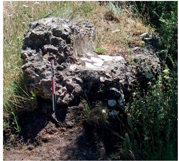
Fig. 6. Aspect of another section of the commonly called Amadora aqueduct, in Gargantada zone (photo José Manuel de Mascarenhas).
