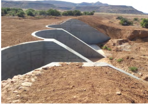
Photo 3. Typical concrete multi-arch weir.
