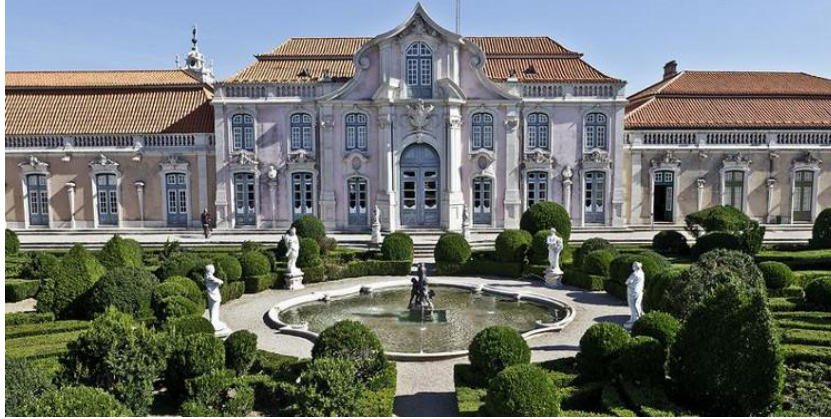
Figure 15. Garden of Malta in Lisbon, Portugal
