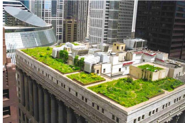
Figure 21. Chicago City Hall Rooftop
