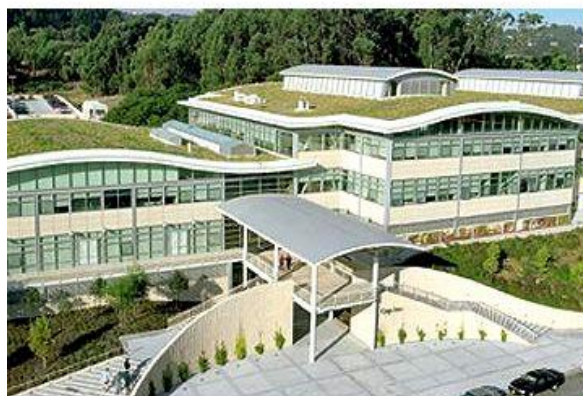
Figure 8. The roofs on the building on the corporate campus of Gap, Inc. in California
