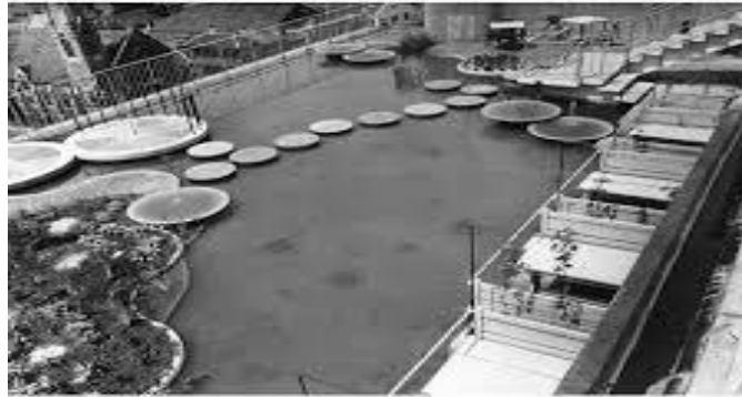
Figure 19. Harvey's Department Store rooftop Garden
