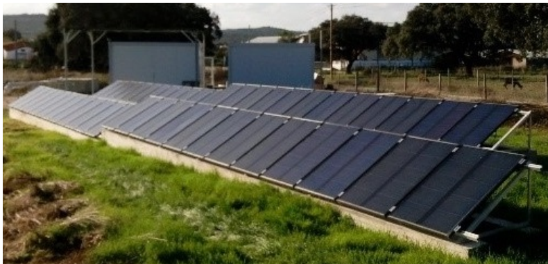
Figure 4.4: Photograph of the PV plant, mounted in the ground near the LIB prototype site (right container behind the PV plant).
