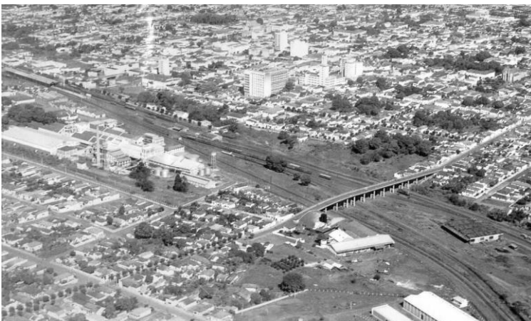
Image 44 – Viaduct “Leonardo Barbieri”, photo from 1965. It connects Vila Xavier to downtown. Source: VALE, Ana Rute, p. 118.
