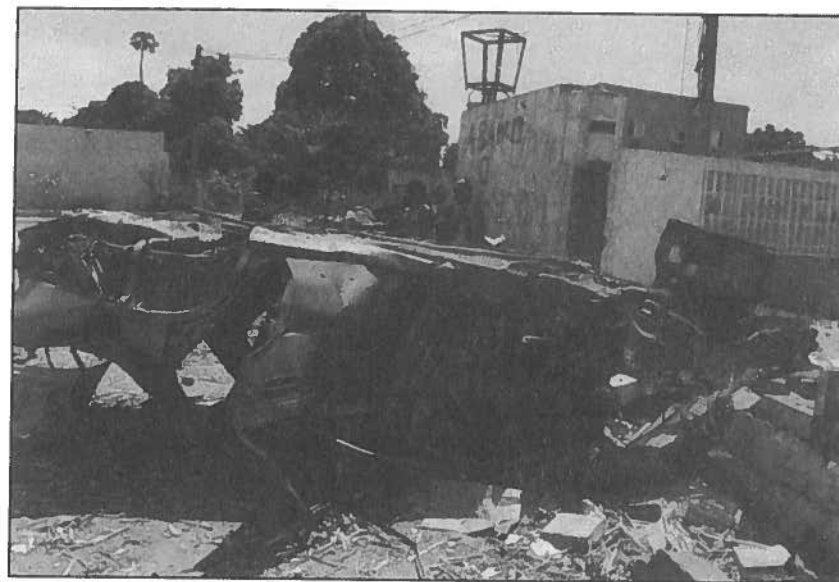
Destruction caused by UNITA in Caxito.
