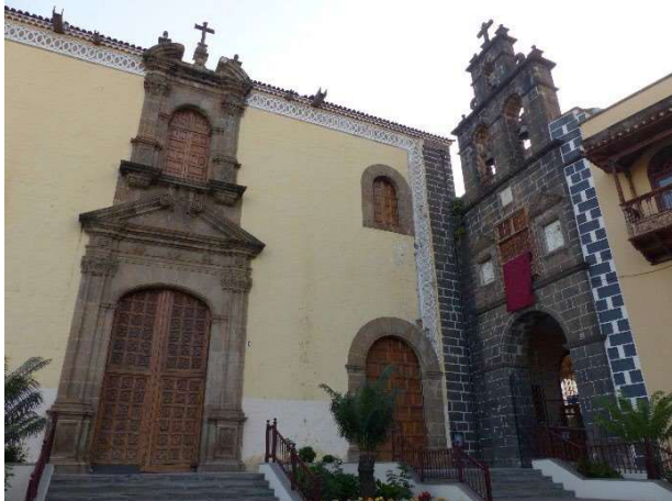
Fig. 3 Main façade of the convent of “San Agustín” (La Orotava)
