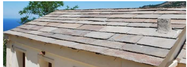
Fig. 5. Slate roof in Ikaria.
