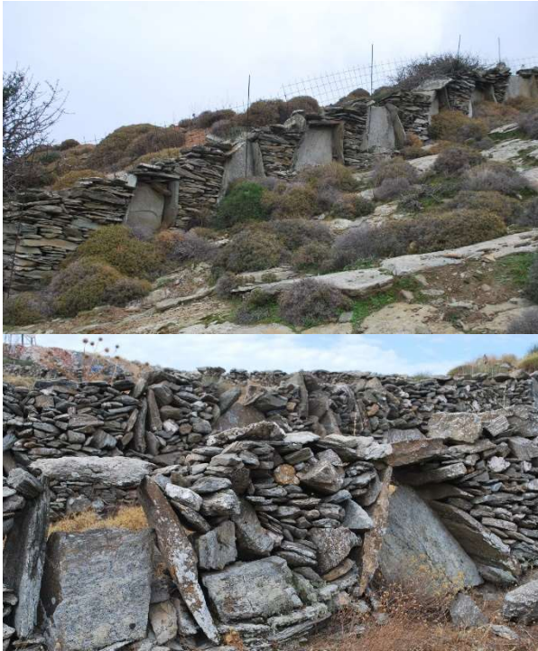
Fig. 2. The art of drystone walling in Andros and Kythnos.
