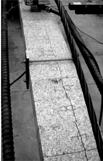
Figure 35: Transversal reinforcement applied to prevent progression of long axial crack and buckling of the sup-pillar.
