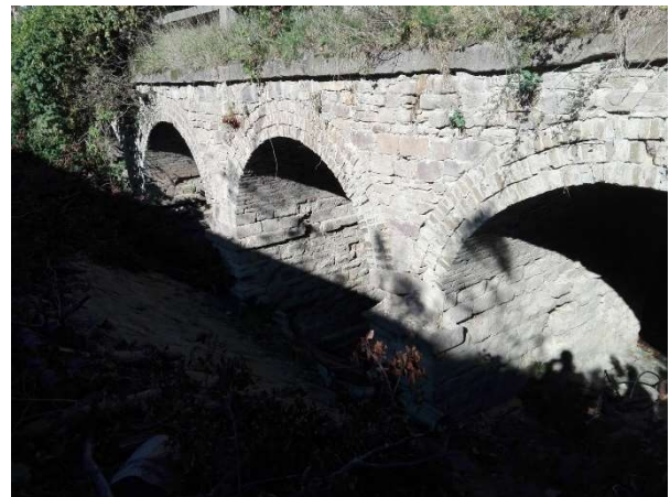
Fig. 2. Bridge of Piliscsaba seen from the north
