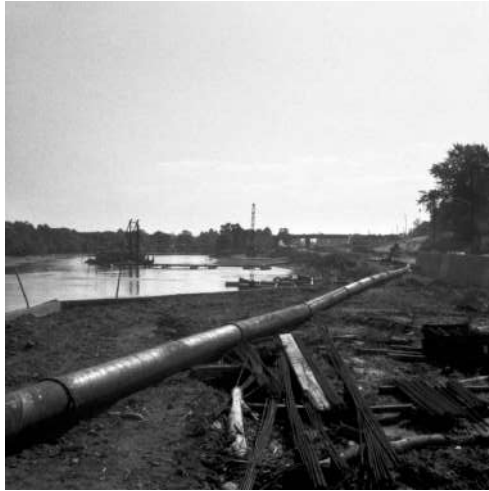
a. The Great Pipes Monument
