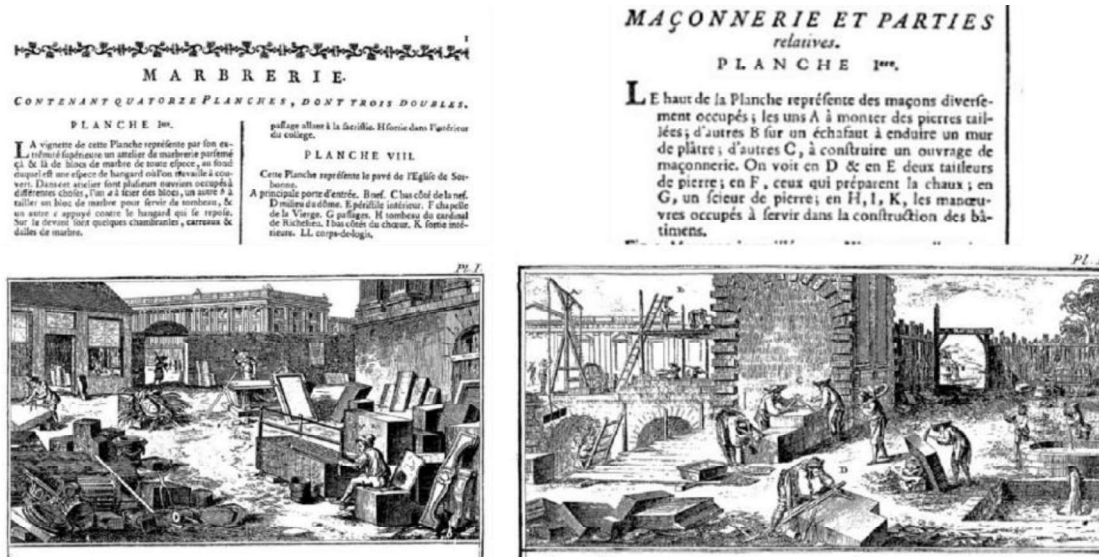
Figure 14 Left: Engraving of a marble transformation and cutting workshop. Right: Engraving of a construction site and representation of the masonry. (Source : Encyclopedia, Diderot, D'Alembert)
