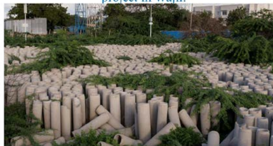
Pipes meant for a massive, incomplete sewage project in Wajir.
