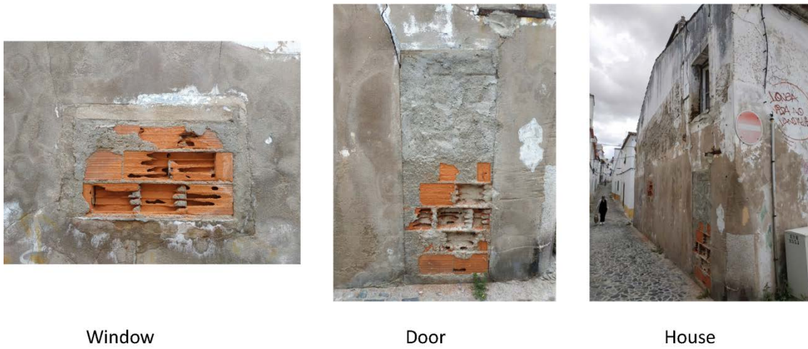
Figure 5.34: Openings of dilapidated houses are closed while they are either abandoned or not being renovated (source: author)
