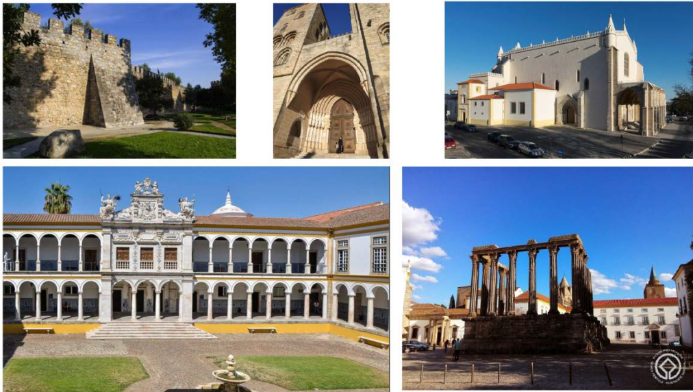
Figure 5.3: Remarkable Historic buildings of Évora (source: author and Google street view)
