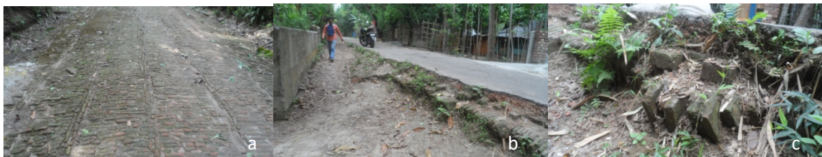
Figure 4.7: (a) officially discovered and preserved the road or highway of Khan Jahan. (b) metaled road constructed by LGED 14 over ancient Khan Jahan road (c) bricks found under the metaled road, possess features similar to that of protected structures.
