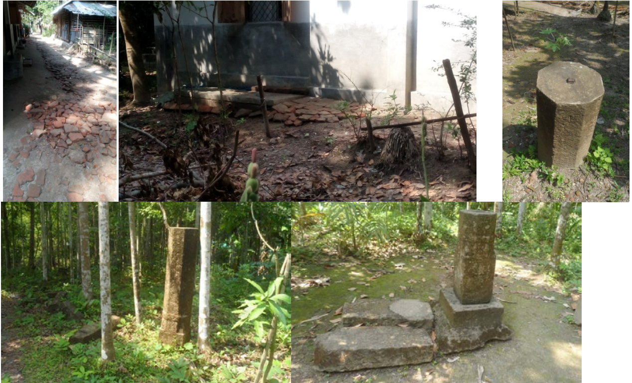
Figure 4.5: The site of Boro Adina Mosque is looted and the historic square shaped bricks are used for making pavement by immediate neighbouring houses ignoring the law and regulations (photo: author).
