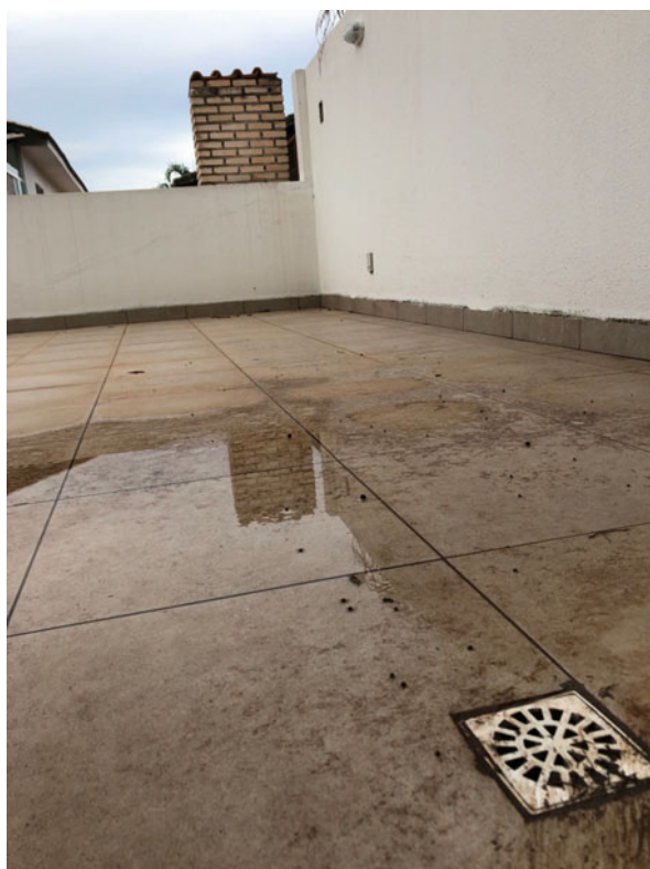
Fig. 5 Terrace for rainwater harvesting in a Brazilian house (Brasilia, central Brazil), inspired by the cistern of Monsaraz village (Alentejo region, Southern Portugal)
