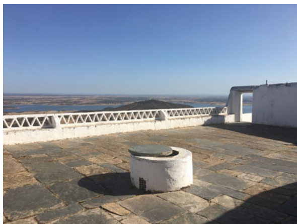
Fig. 3 Terrace for rainwater harvesting above the cistern of Monsaraz village, Alentejo region, Southern Portugal
