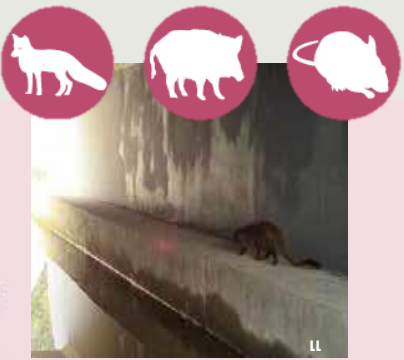
Culverts with dry ledges
