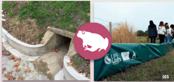
Permanent concrete barriers / temporary canvas barriers
