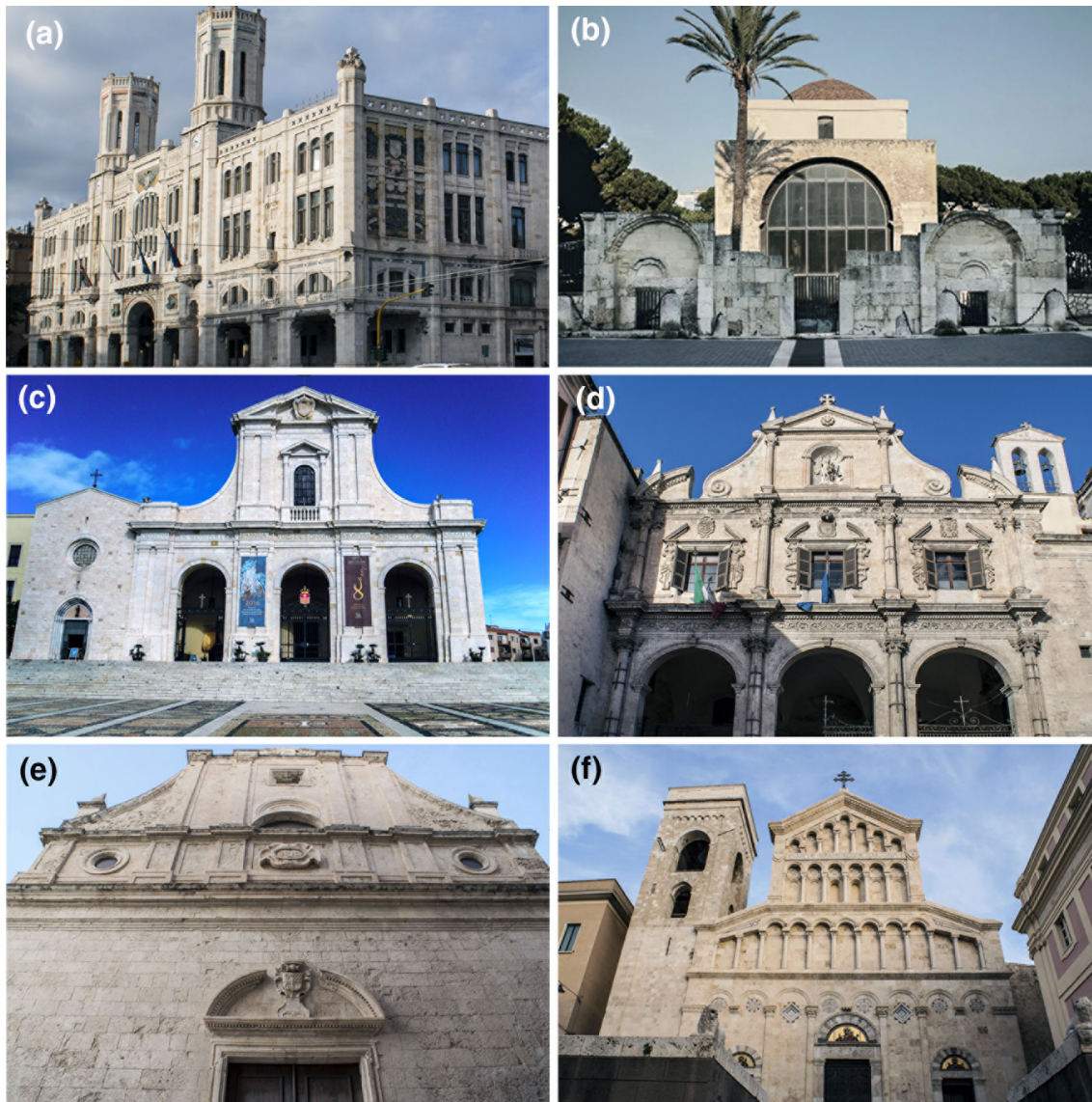
Fig. 2 a Town Hall of Cagliari. The Pietra Forte building stands on a Sardinian granitic plinth (1899–1915); b facade of the San Saturnino Basilica built in 304 AD with the Pietra Cantone limestone. The church was founded originally as a martyrium in honour of the Saint Saturnino Patron of Cagliari; c Façade of Nostra Signora di Bonaria , Sanctuary dated 1704 built with the Pietra Forte ; d San Michele church (1664–1712 AD). The façade is built with
