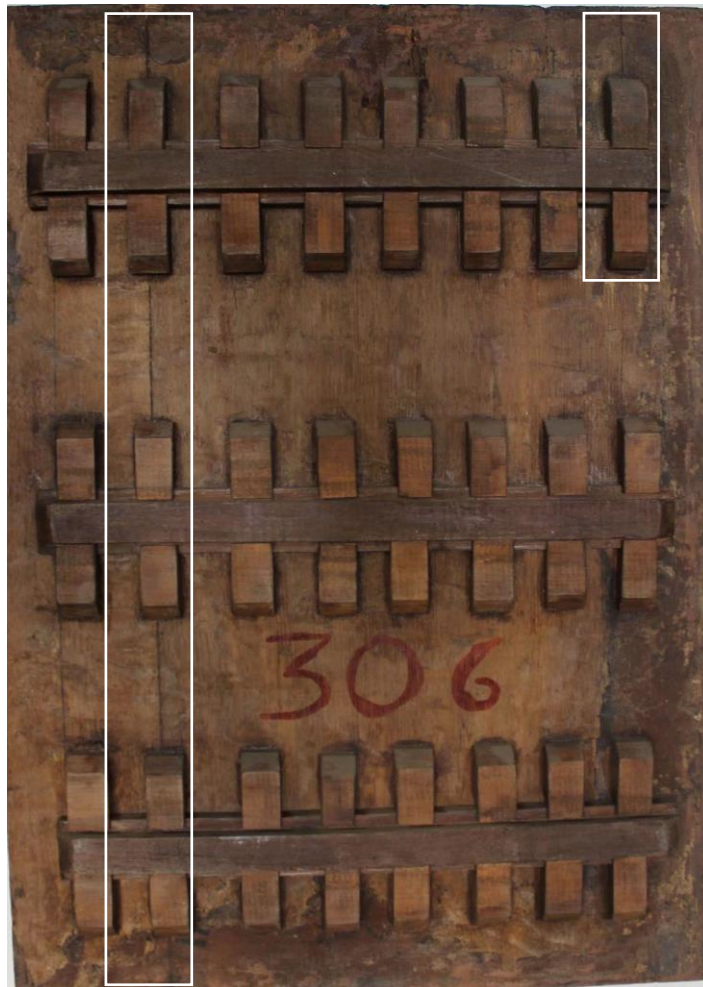
Fig. 12. Images showing the cracks are coinciding with the horizontal parchettatura
