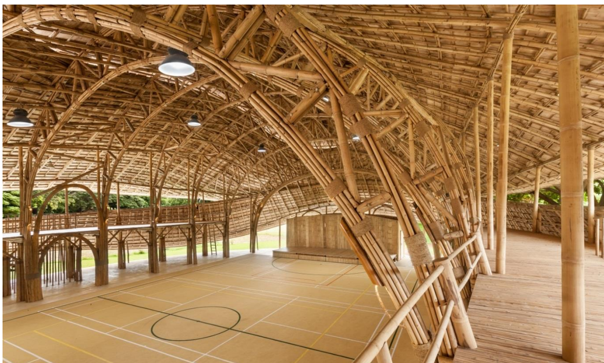
Figura 100 Balcones Laterales Bamboo Sports Hall
