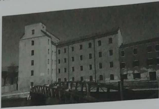
Figure 3. Passuello e Povera Mill. Exterior view from the Valeria Solesin bridge. Venice (Italy). Photo by: Sheila Palomares Alarcón. 2017.
