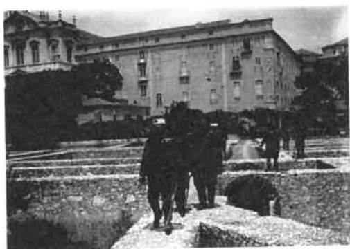
Figure 3. King D. Carlos visiting the Liceu Passos Manuel construction site (1907). Photograph by Joshua Benoliel, Lisbon Municipal Archive, Cod. PT/AMLSB/JBN/000390
