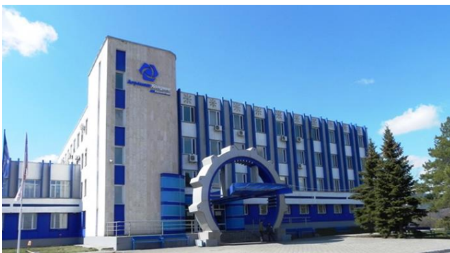
Fig. 16. Administration building of Diesel plant
