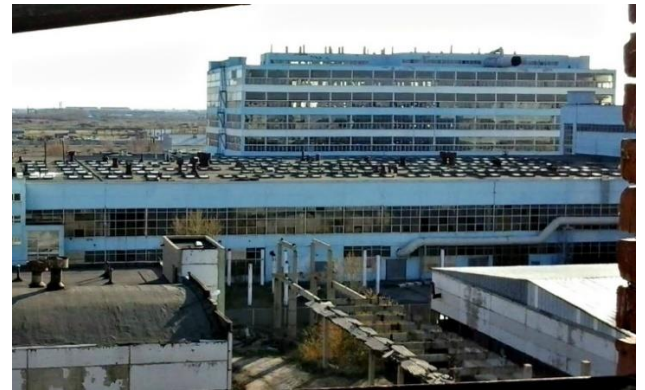
Fig.21. Half restored by “Kazneftehim” corpus of the former Chemical industrial complex. Source: Author
