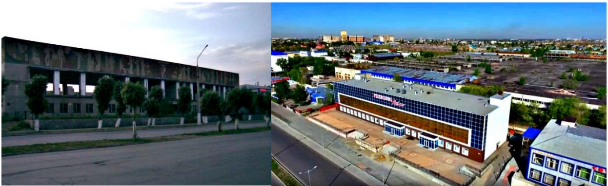
Fig.23. One of former the administrative buildings in 2009 and its reconversion to the Restaurant “Premium Palace” (the former industrial complex is behind).
