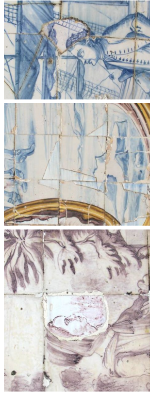
Figures 2 to 4. Three examples of replacement of missing fragments with modern glazed ceramic fragments made on purpose.
