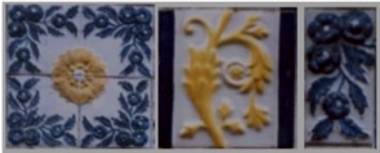
Image A.21 – The embossed tiles that covered the façade of Frontaria Azulejada House, Santos, Brazil
