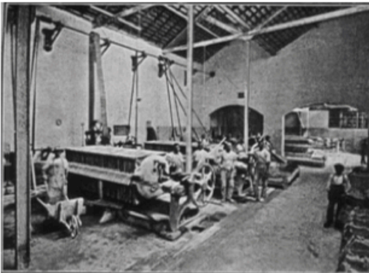
Image A.132 – Interior image of The Santa Catharina Factory – Section of Crushing and Milling (FABRICA SANTA CATHARINA – Fagundes, Ranzini & Cia.)
