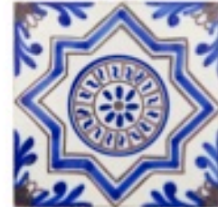
Image A.30 – image of the Dutch pattern of tile used in the façade of the building.
