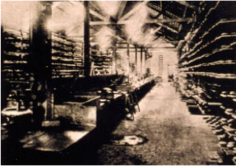
Image A.134 – Interior image of The Santa Catharina Factory – Section of lathes benches for making empties and also, in the center of the image, a glaze mixer and a glazing pond (FABRICA SANTA CATHARINA – Fagundes, Ranzini & Cia.)
