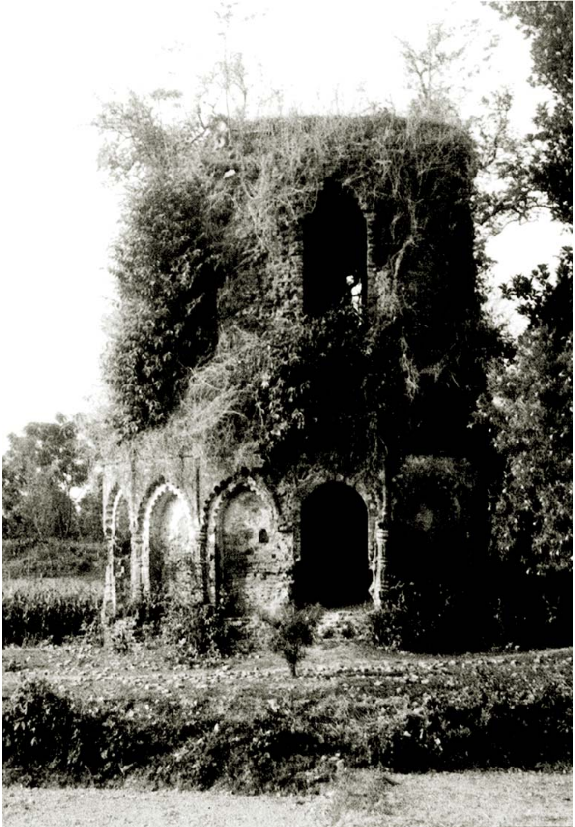
Figure 12: Most of the historical excellences have gone with the nature by the passage of time and as mud, sun dried brick and the burnt brick originated by clay, so temporariness in the structure and mostly for the moisture and saline factors Photo Source: Sajid Bin DOZA
