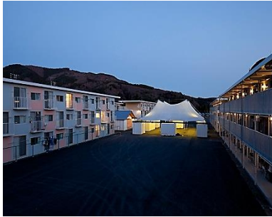
Figura 190 –Onagawa Container Temporary Housing. (Hiroyuki Hirai)
