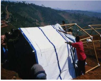
Figura 177 – Paper Emergency Shelter para UNHCR. (Shigeru Ban architects)
