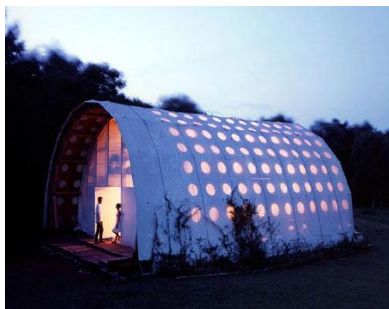
Figura 179 – Aspecto exterior do projeto Paper Studio - Keio University, Japan, 2003. (Shigeru Ban architects)
