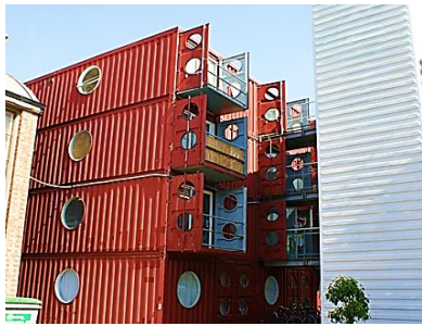
Figura 225 – Container City I
