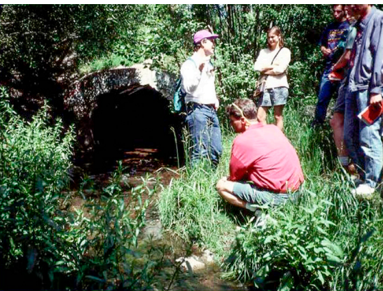
Figure 4 – Strawberry Creek emerges from an underground culvert in Berkeley, California. The creek was exhumed from the pipe in the 1980s, an early and influential example of urban stream “daylighting”. (photo by author, 1992)
