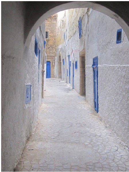
Figure 5 – Repair work in a street of the old medina in Safi, organised by JEC and IRMSS. Photo by JEC, June 2015
