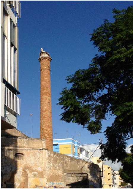
Figure 6 – Old brick factory chimney surrounded by modern buildings, hosts a stork's nest
