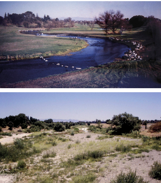
Figure 9 – Uvas Creek, Gilroy, California. View downstream from Santa Teresa Boulevard bridge. (a) in January 1996, two months after a channel reconstruction project, showing symmetrical meanders, with outside bends protected by boulders and log revetments, typical of such projects. (b) the same view in July 1997, after a modest flood (return interval about 6 years) washed out the reconstructed channel, reestablishing a form more typical for its Mediterranean-climate setting. (from Kondolf, Smeltzer, and Railsback, “Design and performance of a channel reconstruction project in a coastal California gravel-bed stream,” Environmental Management , 2001)
