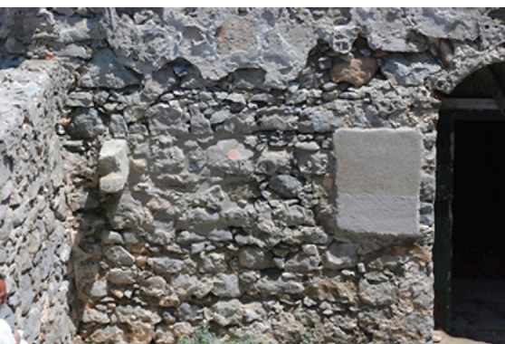
Figure 8 – Joint treatment and wall coating plaster tests
