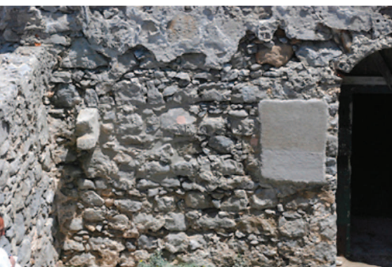
Figure 8 – Joint treatment and wall coating plaster tests
